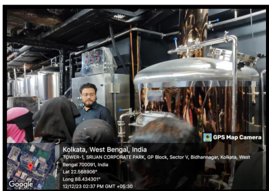
Mr. Rahul Roy (Assistant Brewer) explaining the structure and working of fermenter.
